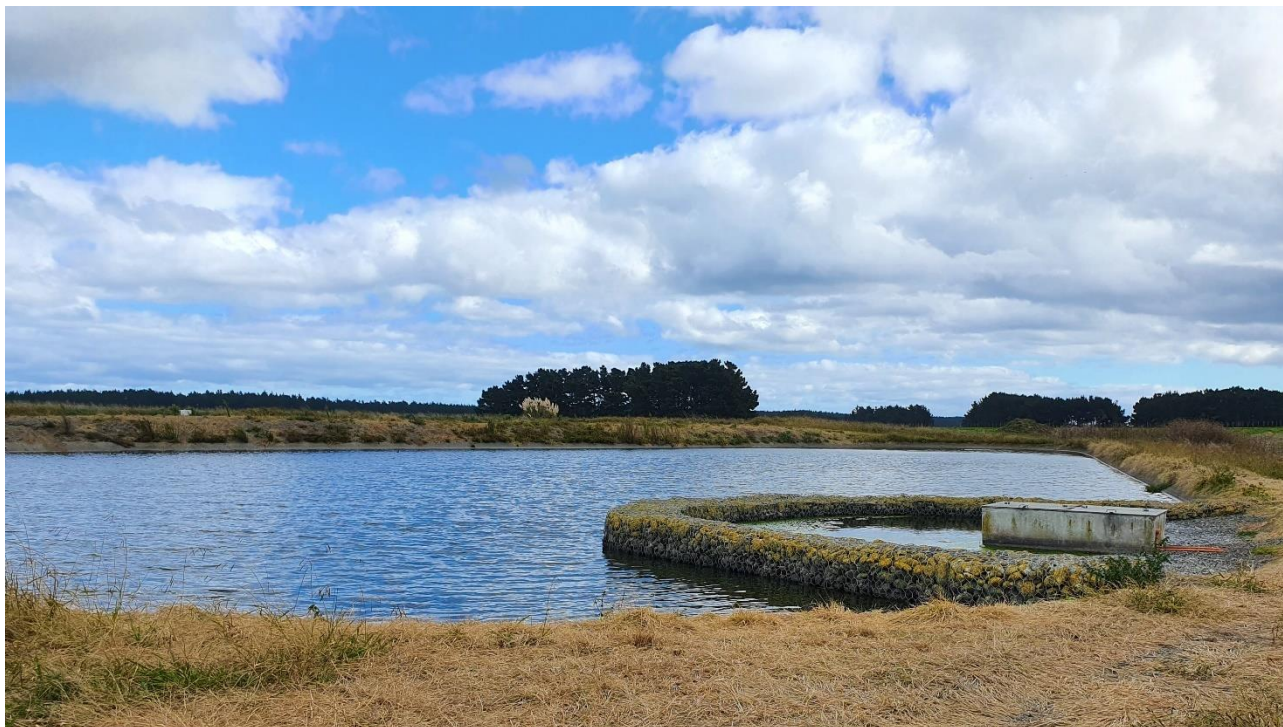
Figure 5-5: Ratana WWTP Pond 2, Outlet Area
