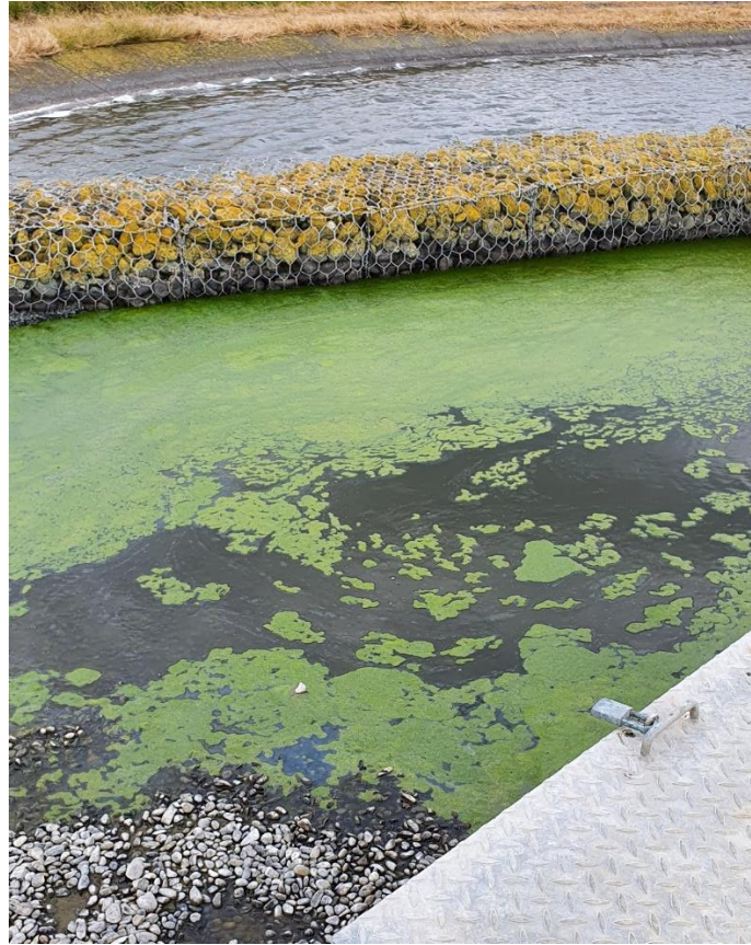
Figure 5-6: Pond 2 Outlet showing gabions, gravel, and overflow chamber
